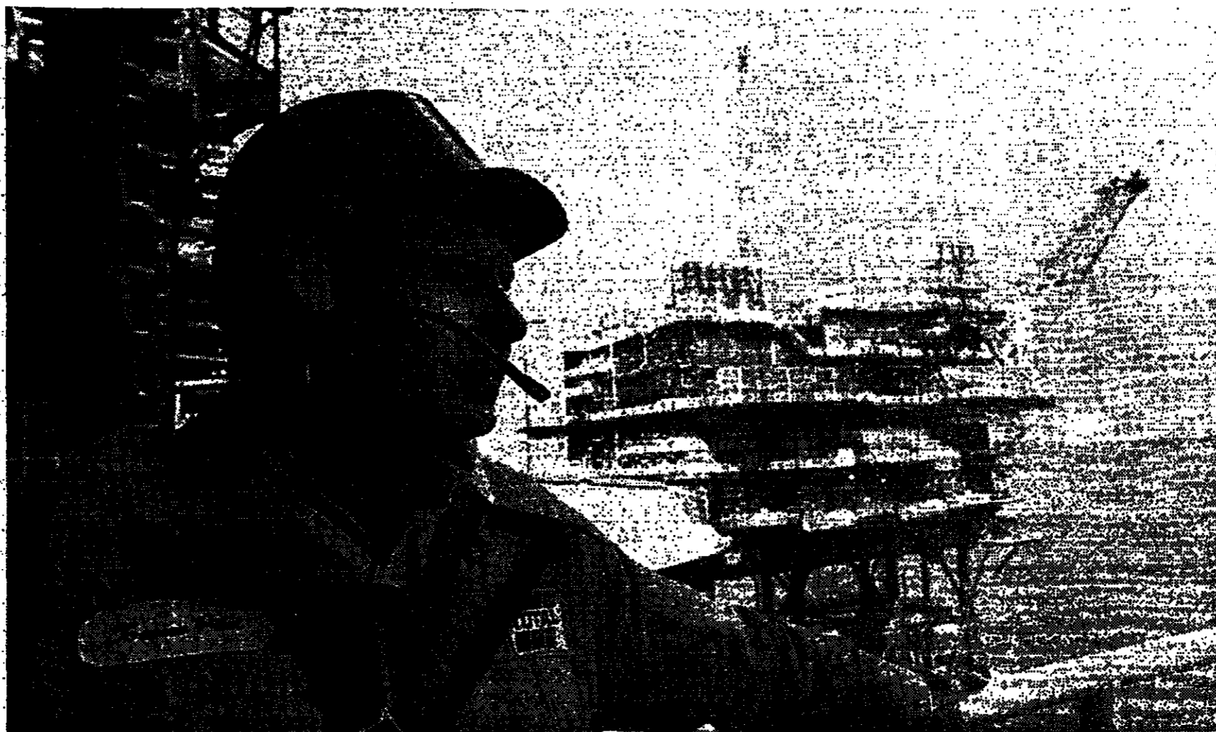
Total Oil Marine's Alwyn Field platform in the North Sea
